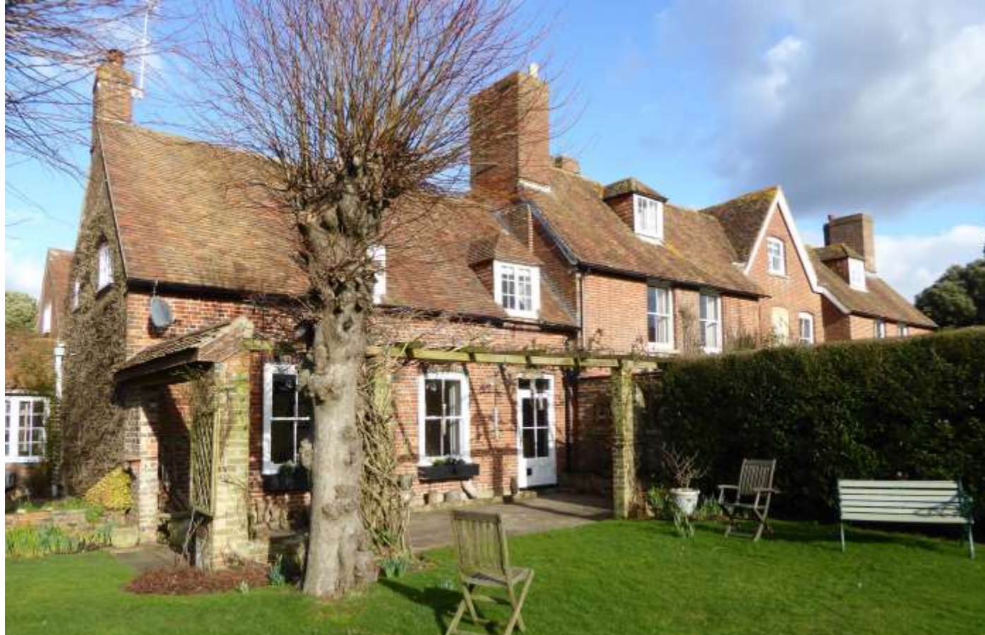
Plate 5: Oblique view of the south façade of Great Posbrook from the south-west (the garden of Old Barn Cottage).
