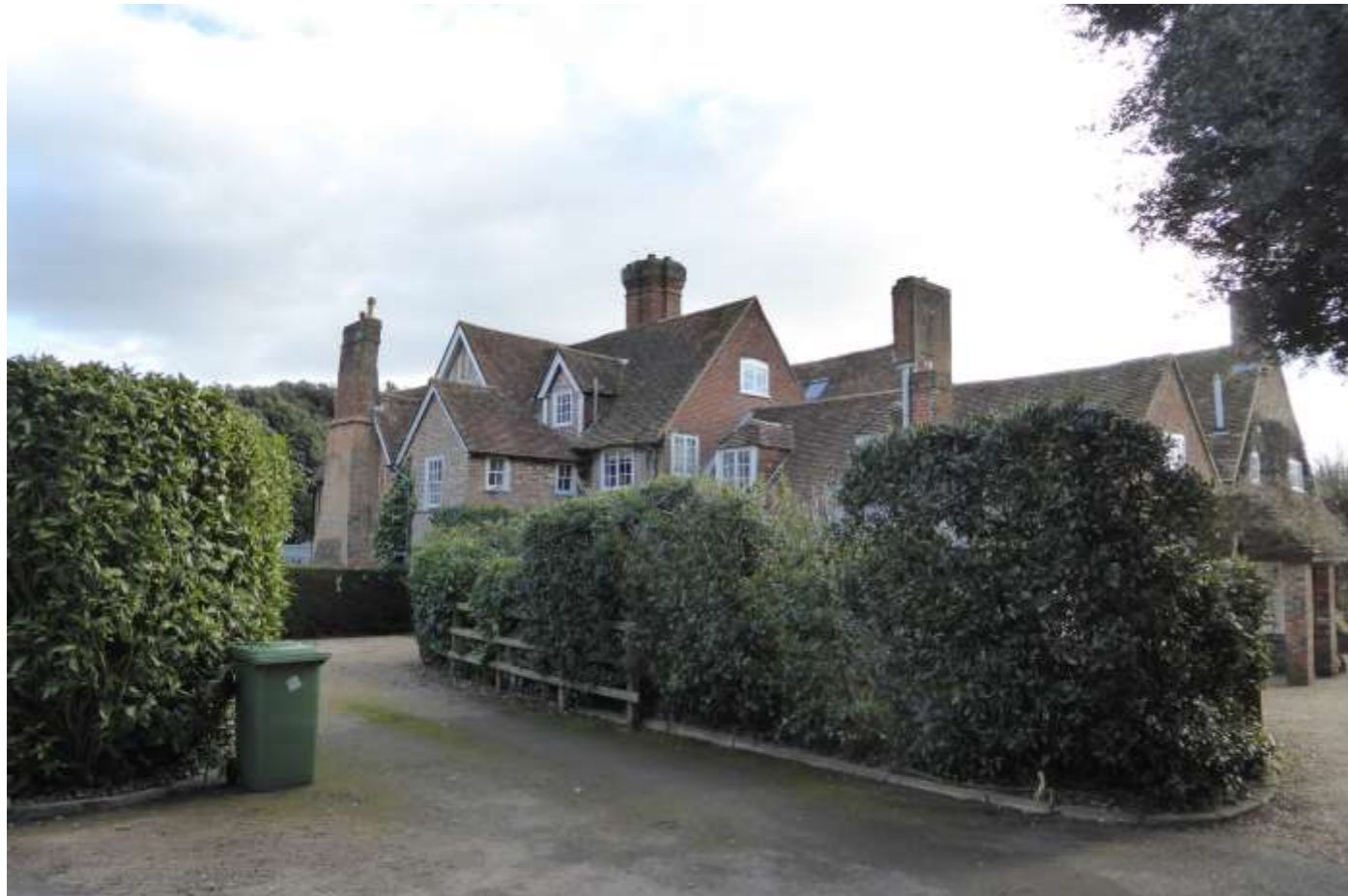
Plate 2: Great Posbrook, from the entrance drive to the Middle House.
